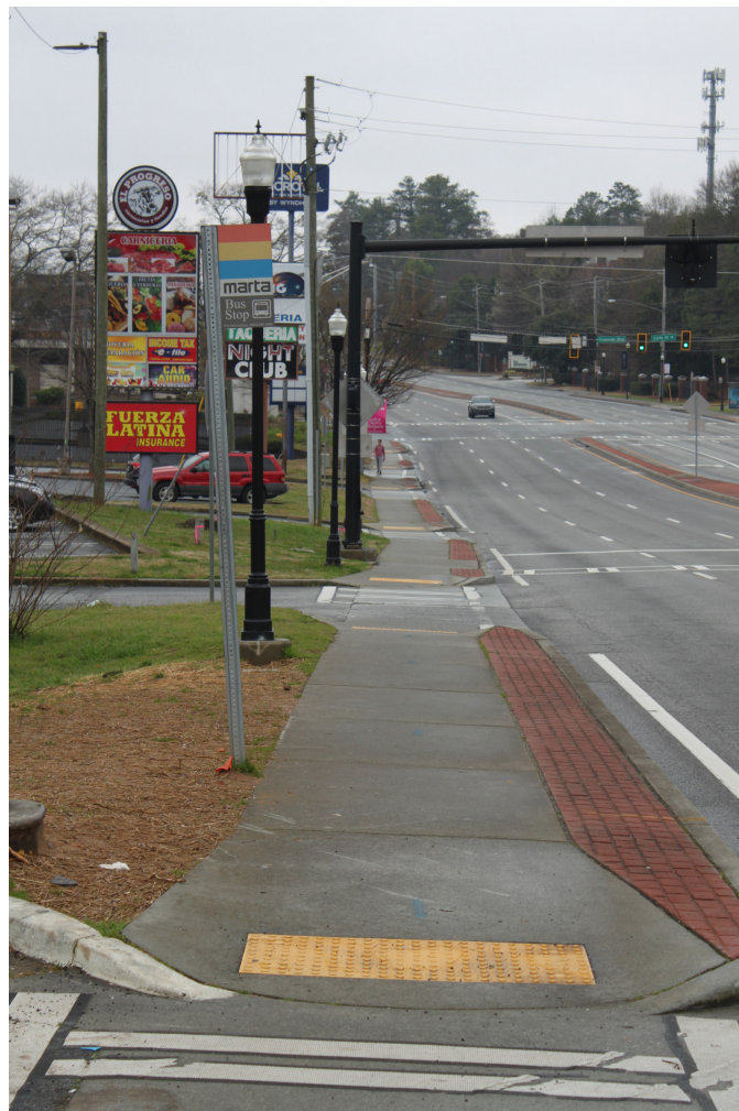
Newly completed signalized mid-block crossings are a safety upgrade in the corridor area.
