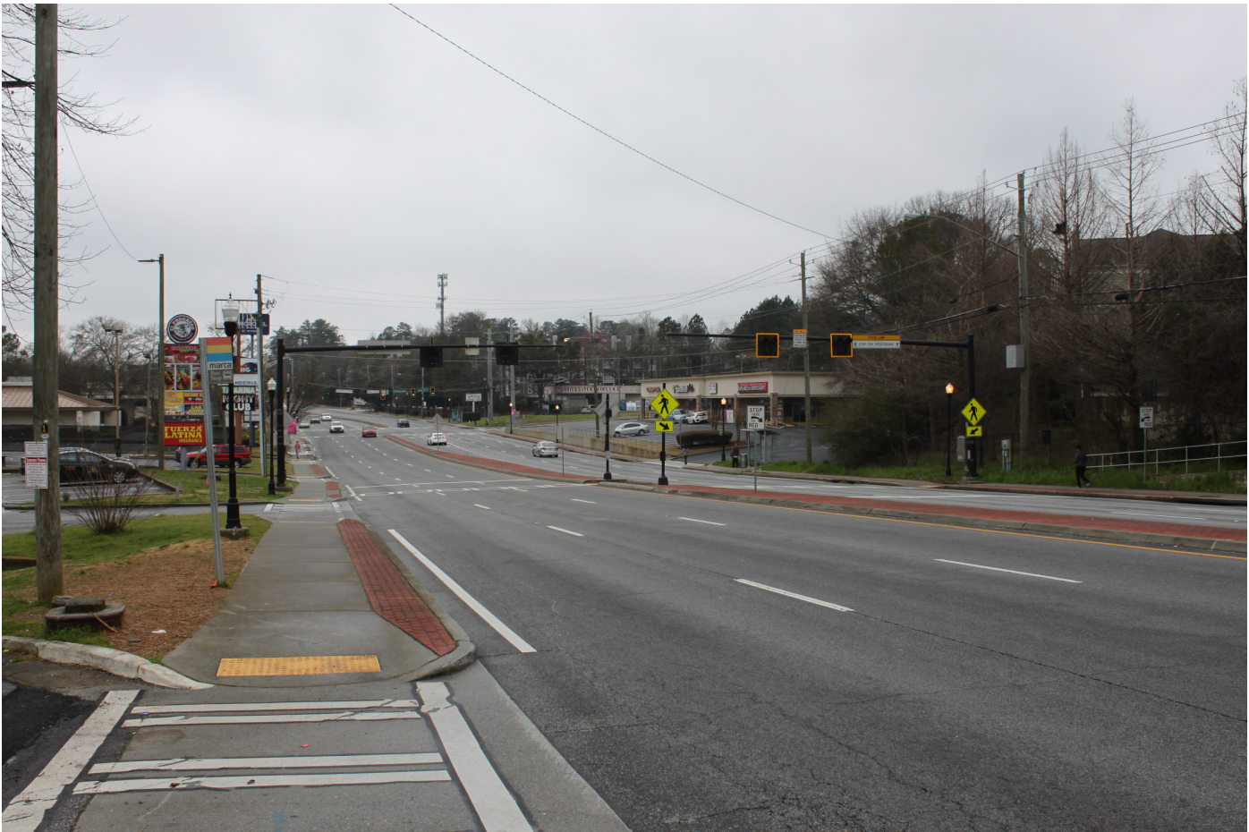
The Buford Highway Corridor includes many new pedestrian amenities since the 2014 study including midblock crossings with HAWK signals, new crosswalks at driveway cuts, and accessible sidewalks.
