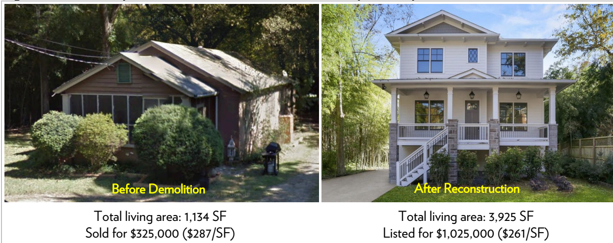
Figure 6: Case Study of Tear Down-Reconstruction Activity, 1404 Sylvan Circle
